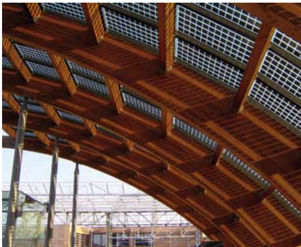
Fotovoltaico integrato Environmental Park (TO)
