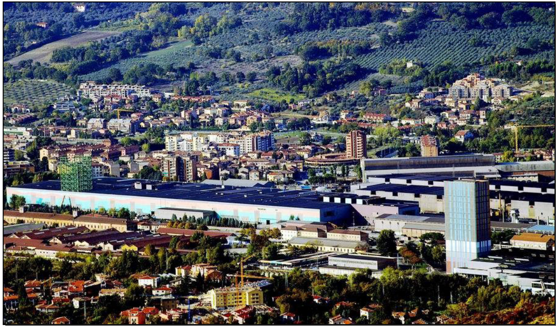
Foto: Pablito_TR - Fabio M. - http://www.flickr.com/photos/pablito_tr/2044074999/
